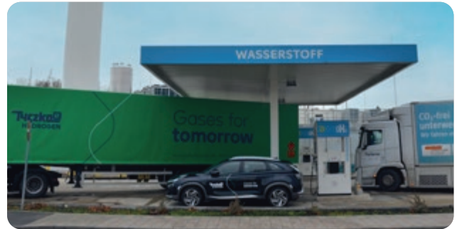
Public refuelling stations
